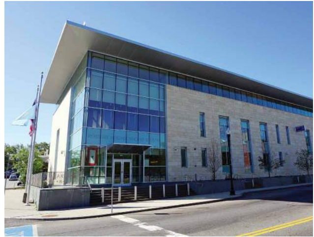
The B-2 Police Station in Dudley Square earned LEED Silver certification with extensive daylighting and a vegetated roof.
