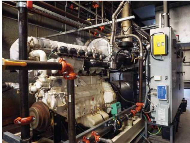
The combined heat-and-power plant at West Roxbury Education Center was upgraded in the summer of 2015. It provides the school with highly efficient heating and power, as well as cooling through the use of absorption chillers. It is configured to be load-following, to further increase system efficiency.
