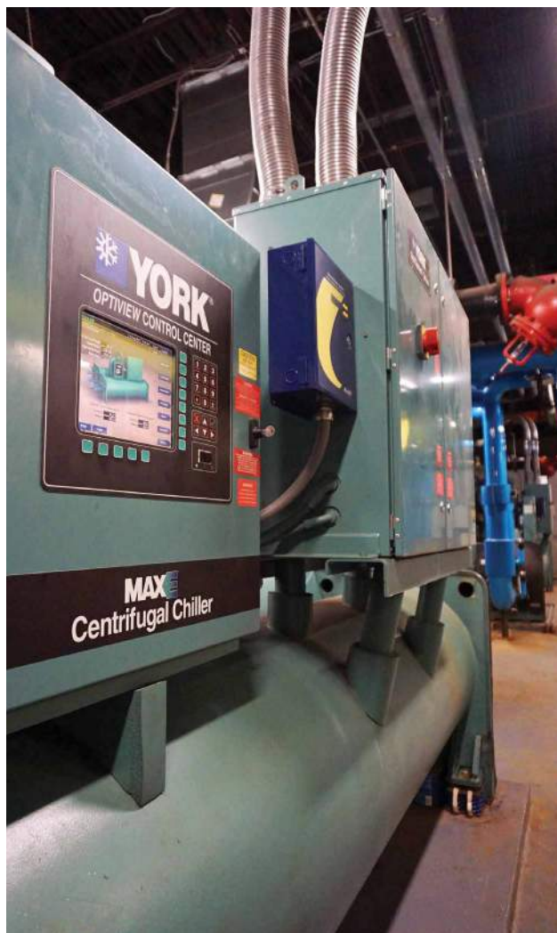
A chiller control panel at West Roxbury Education Center allows for the chiller's operation to be monitored in detail and fine-tuned.
