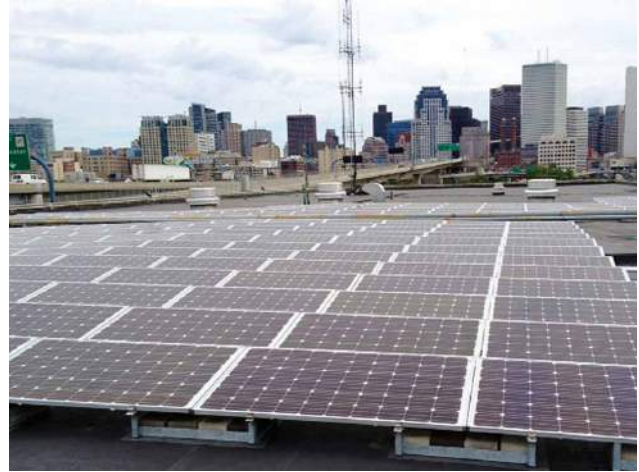
In 2012, the City of Boston installed solar panel arrays on the roof of the Public Works Central Maintenance Facility at 400 Frontage Road. The solar panels power the emergency operation of traffic control systems at eighteen intersections along key evacuation routes.
