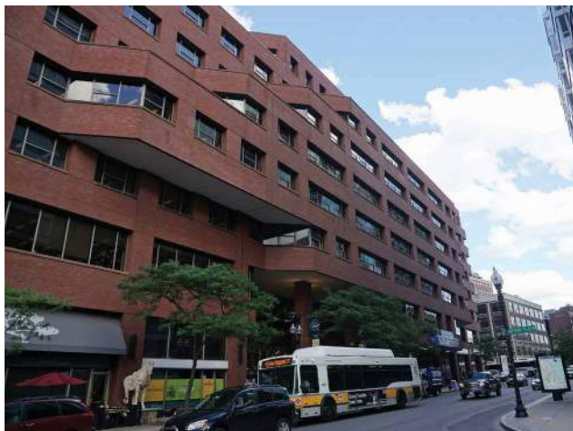
The State Transportation Building uses solar collectors and heat recovered from electrical equipment to supply the building's heating and hot water needs.
