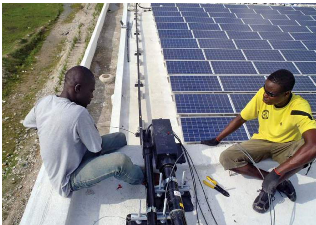
Top left: With 300 beds and six modern operating theaters, University Hospital is the largest solar-powered hospital in the world that produces more than 100 percent of its required energy during peak daylight hours
