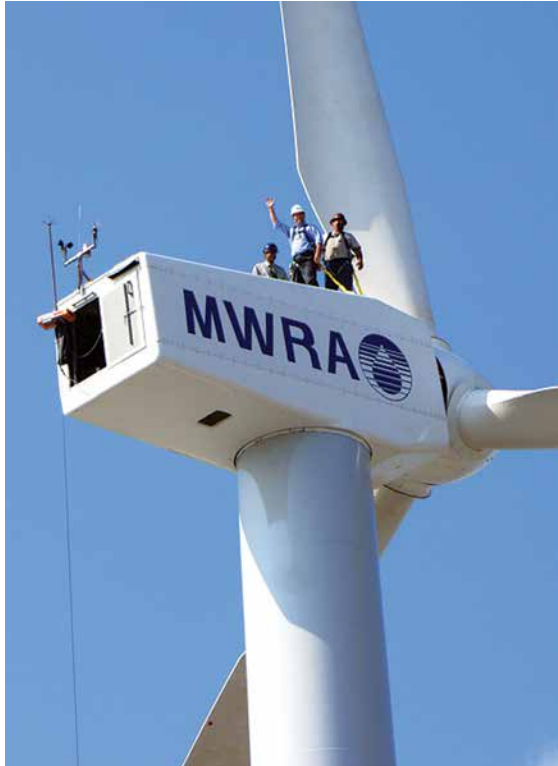
In 2011, a 365-foot wind turbine was installed in Charlestown. It generates 3 million kilowatt hours per year and provides a $300,000 annual savings in electricity costs. The project was funded through the American Recovery and Reinvestment Act (ARRA).
