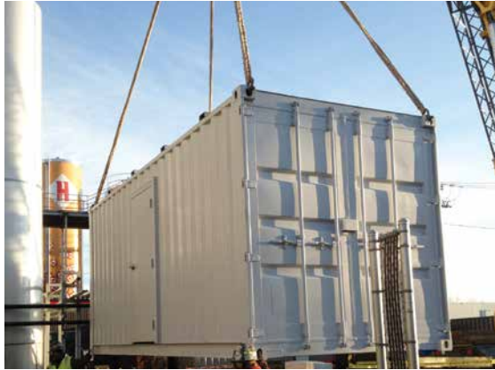
In 2013, Harpoon Brewery installed a co-generation system at their Boston Brewery to simultaneously generate electricity and heat.
