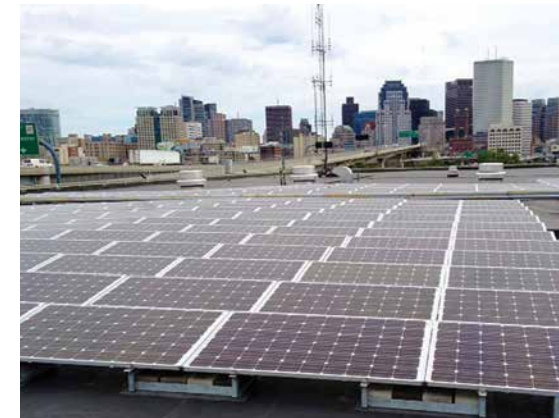
In 2012, the City of Boston installed solar panel arrays on the roof of the City Public Works Facility to apply green technologies to power the emergency operation of traffic control systems at 18 intersections along the City of Boston's evacuation route.
