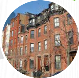
BAY VILLAGE Cortes St.
